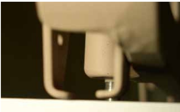
Carefully inspect the seat feet per Cessna service bulletin SEB 11-4 and NEB11-2
